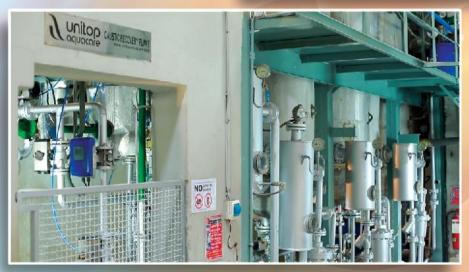
**CRP:** Its Caustic Recovery Plant recovers about seventy percent of the caustic soda used in mercerizing of fabrics. Plant's capacity is 4.5 tons per day. This recovered soda is reused it in the process again and again, continually.
